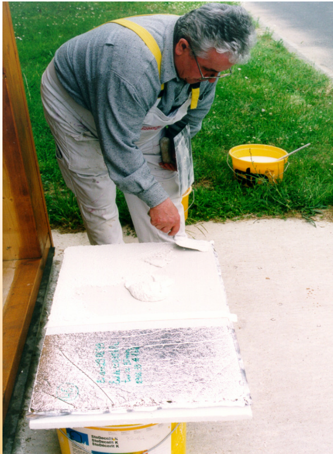
application of plaster
