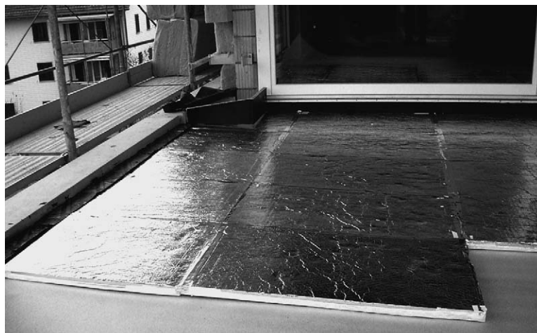
Fig. 2. VIP insulation of a terrace with heated rooms beneath. The panels are placed on a thin polystyrene foam layer for mechanical protection.
