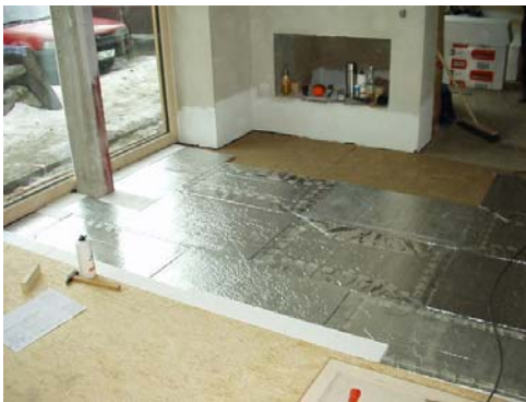
Figure 67: Left: Photo taken during renovation. The OSB can be seen in the foreground, the VIP in the centre and the softboard in the background. (foto: may.schurr.architekten, Bad Wörishofen) Right: Cross-section of the floor set-up
