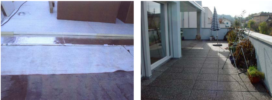
Figure 29: Building site – finished terrace: VIP is already well protected during installation.
