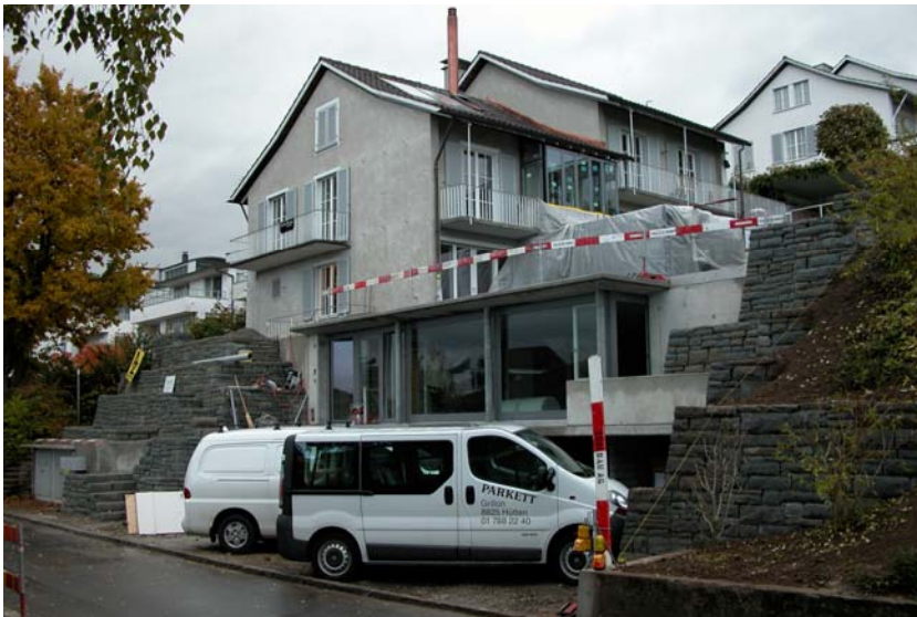
Figure 19: Single-storey studio construction in the embankment above open garage and below walk-on terrace
