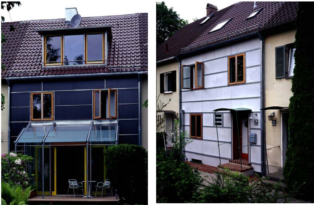
Figure 47: South and north façade after renovation
