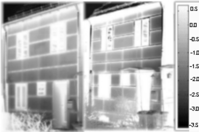
Figure 50: Infra-red images of the north side of the building On the left: 2002, on the right: 2003
