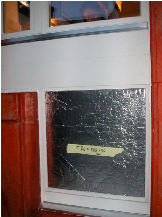
Figure 36: Window element with tight-fitting VIP
