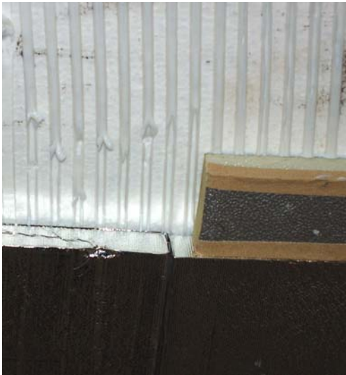
Figure 52: Left: Installation of the VIP with dispersion based mortar onto the polystyrene boards. The horizontal strips of polyurethane can be seen as well as the vertical strips of dispersion based mortar.
