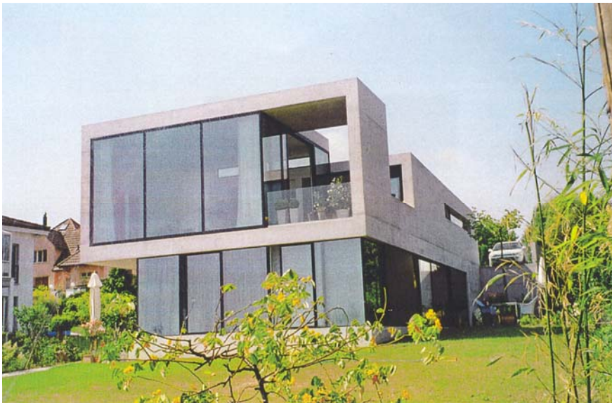
Figure 32: Single-family house with VIP-Multiplac wall elements
