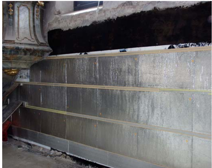
Figure 52: Left: Installation of the VIP with dispersion based mortar onto the polystyrene boards. The horizontal strips of polyurethane can be seen as well as the vertical strips of dispersion based mortar.
