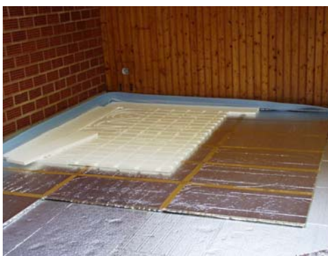
Figure 69: Left: Photograph of the floor during the installation. The shiny VIP are put on the matt aluminium layer of the polyurethane boards. The VIP were connected with tape. White polystyrene plates with grooves for the heating pipes are mounted on top of the VIP. Right: Cross-section of the floor insulated with polystyrene as well as with VIP
