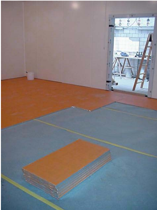
Figure 30: Building site of the floor insulation
