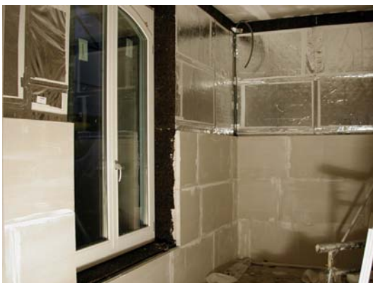
Figure 25: Left: Interior VIP insulation with gypsum board walling in front Right: Finished dormer window
