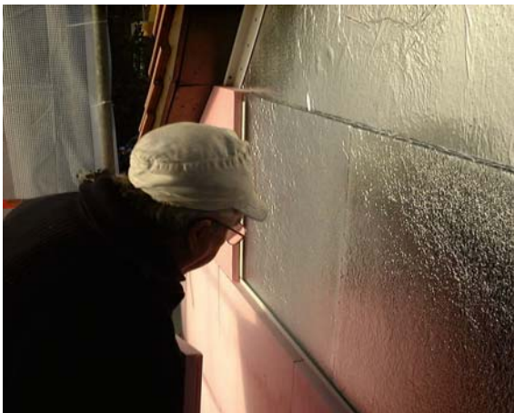
Figure 41: Gable during installation. The shiny VIP are already in the rail system. The pale pink polystyrene boards are being mounted.
