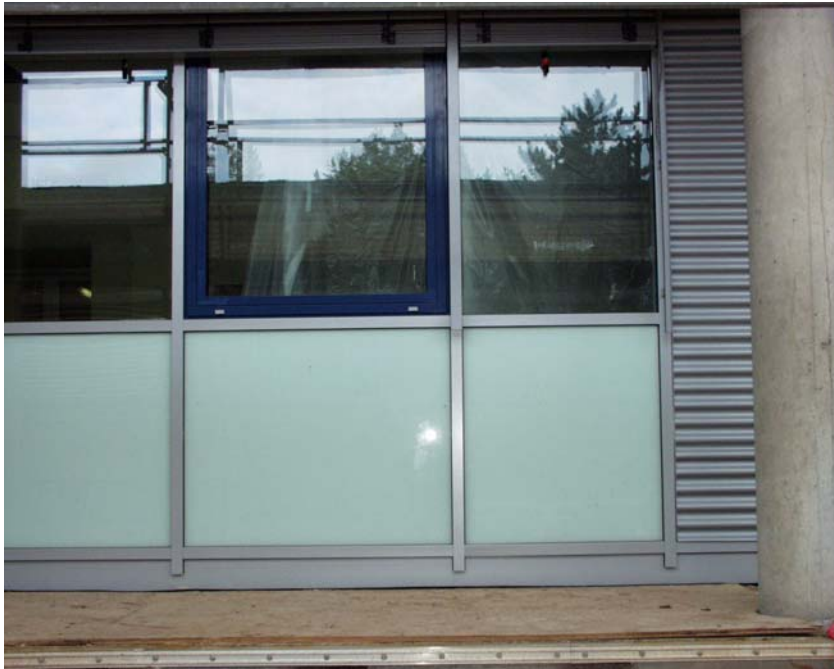
Figure 53: Outside view of the façade
