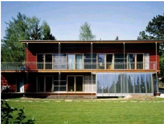
Figure 43: Left: South view of the house. Vertical collectors are integrated between the French windows Right: North-east view of the house
