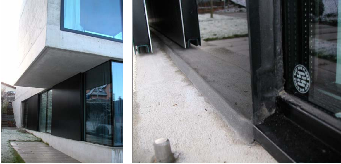
Figure 34: Façade detail with sliding elements in rest position in front of VIP wall elements
