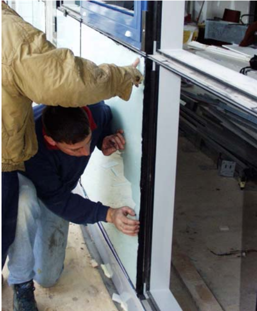
Figure 56: Photograph of the vacuum-insulated façade elements being installed
