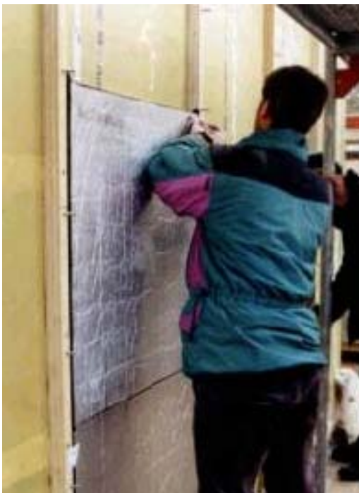
Figure 45: Installation of the VIP into the lath construction
