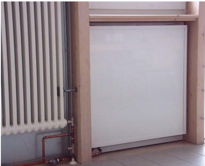
Figure 58: View of the integrated façade system from inside the room
