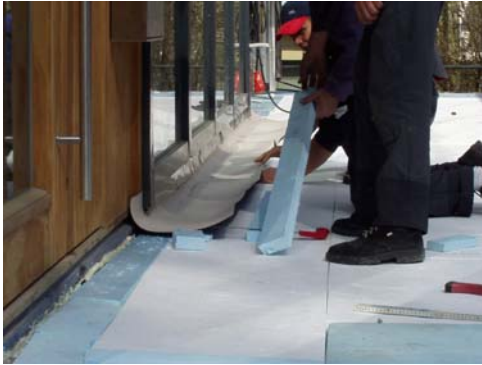
Figure 66: Left: Installing the polystyrene-encased VIP. The border between the floor and the house was filled with pieces of polystyrene. (foto: may.schurr.architekten, Bad Wörishofen) Right: Insulation design
